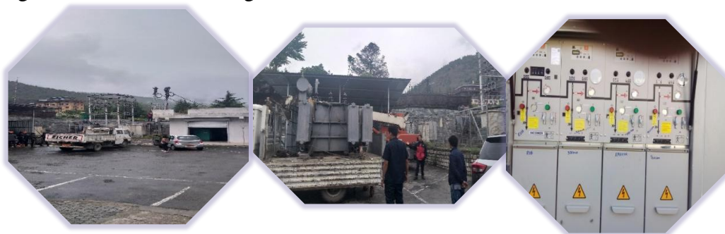
Changing the transformer and installing RMU
